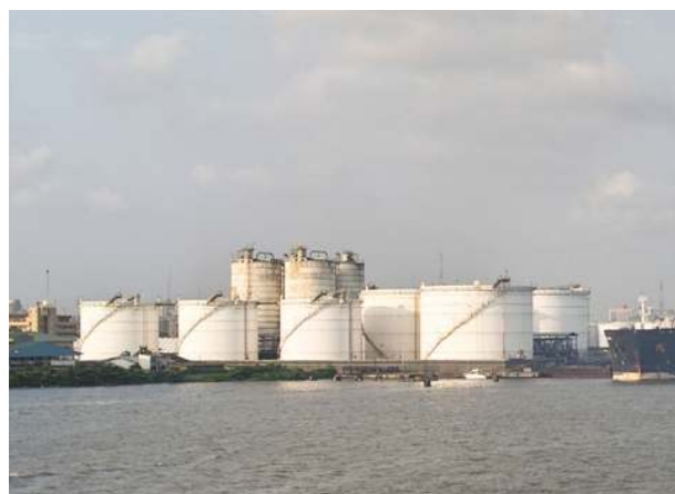
Figure 1.3 A chemical factory in Lagos
