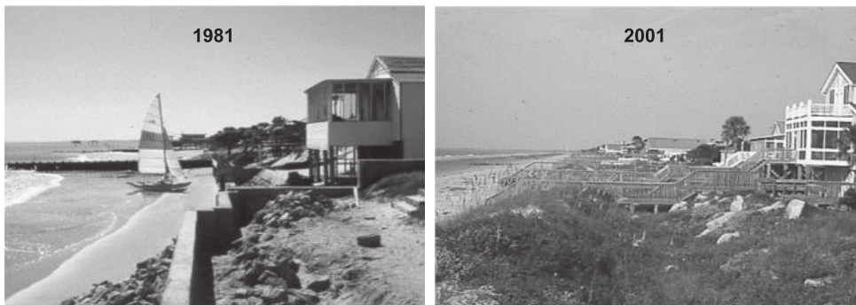
Figure 1.2 Two views of Folly Beach, South Carolina, USA, showing the effect of beach nourishment in reestablishing dunes.
