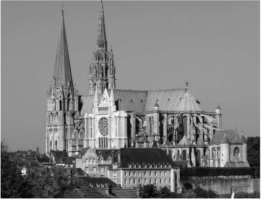
Figure 1.1 Chartres Cathedral, southern façade. The bridge-like structures between the Romanesque tower and the transept (marked by the rose window) and around the rear on the eastern side are the ‘flying buttresses’ supporting the walls.
