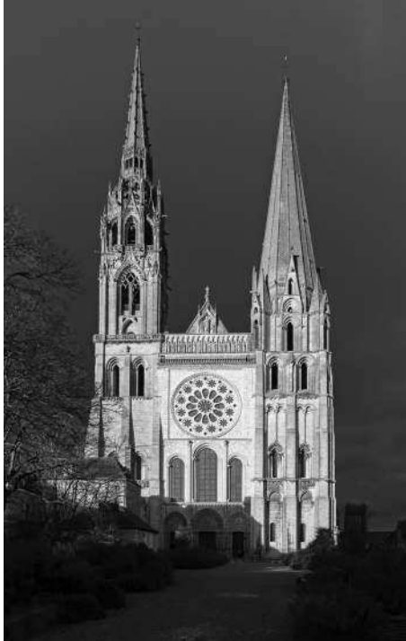
Figure 1.3 The Asymmetrical Reality: the Chartres Cathedral's façade. Note that while the center – built more or less continuously – is properly symmetrical, the two towers, and especially the spires – built some four centuries apart – are growingly asymmetrical.
