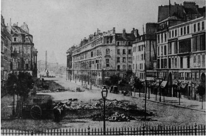
Figure 1.1 Photo taken by Hippolyte Bayard from the steps of the Madeleine late February 1848, looking down the rue Royale toward the Place de la Concorde and the Palais Bourbon. The remains of two barricades are visible in the foreground. Hulton Archive via Getty
