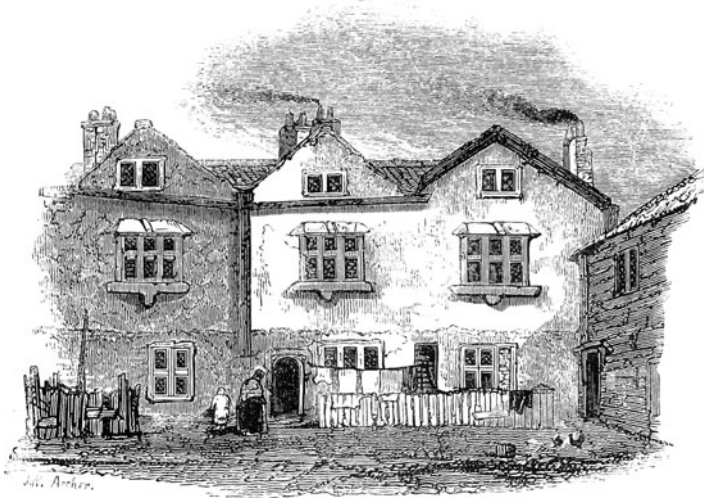
[Existing Remains of the Conventual Buildings.]
