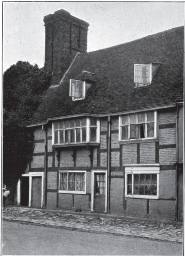
FIG. 10. Houses at Biddenden, Kent. Tile roof swept over oriel window.
