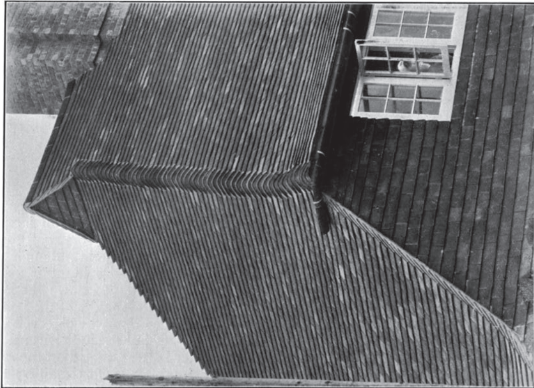
FIG. 3. Gablet, hip and verge treatments.
