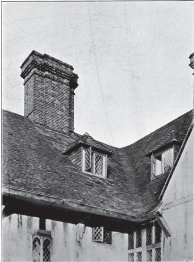
FIG. 20. Swept valley-tiles cut to wedge shapes.
