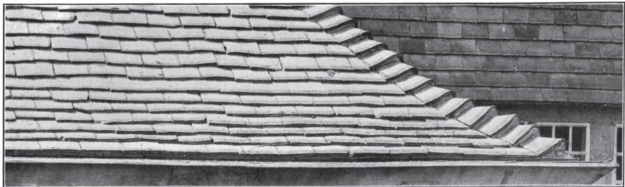
FIG. 18. "Granny" bonnet hip tiles well set up and swept to a good bellcast.
