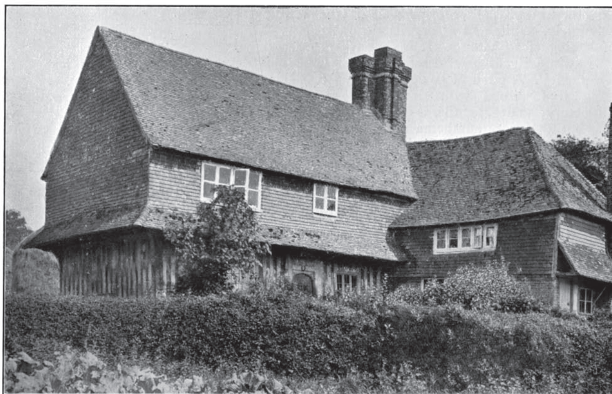
FIG. 2. Kitchingham Farm, Robertsbridge, Sussex. Old-fashioned roof treatment.
