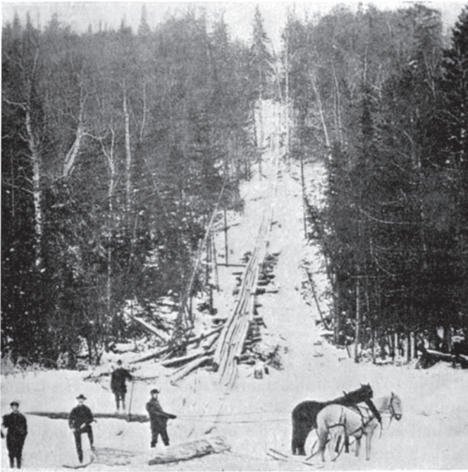
Fig 1. A Log Chute, Canada.
