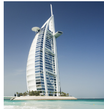
Tertiary sector – the breathtaking Burj Al Arab hotel in Dubai
