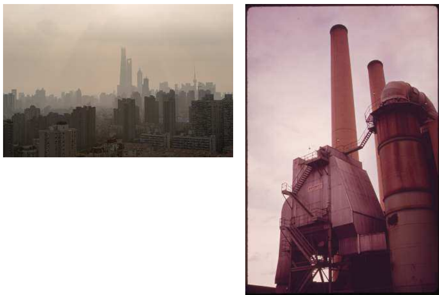
FIGURE 1.12 Smog in Shanghai, China (left) (Wenjie Dong / E+ / Getty Images). Pollution controls are important components of fossil-fueled power plants. Shown here (right) is an electrostatic precipitator, which removes particulate matter from the flue gases of a power plant (nsf / Alamy Stock Photo).
