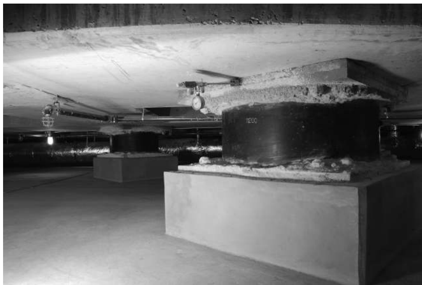
Figure 1.1 Seismic base isolation system under the State Capitol Building in Utah (source: https://commons.wikimedia.org/wiki/File:Base_isolators_under_the_Utah_State_Capitol.jpg )
