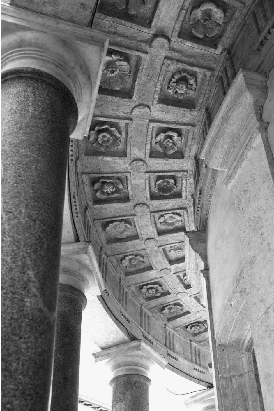
viii. Tempietto. View of soffit and inner surface of entablature. Photo courtesy of Marcello Leotta.
