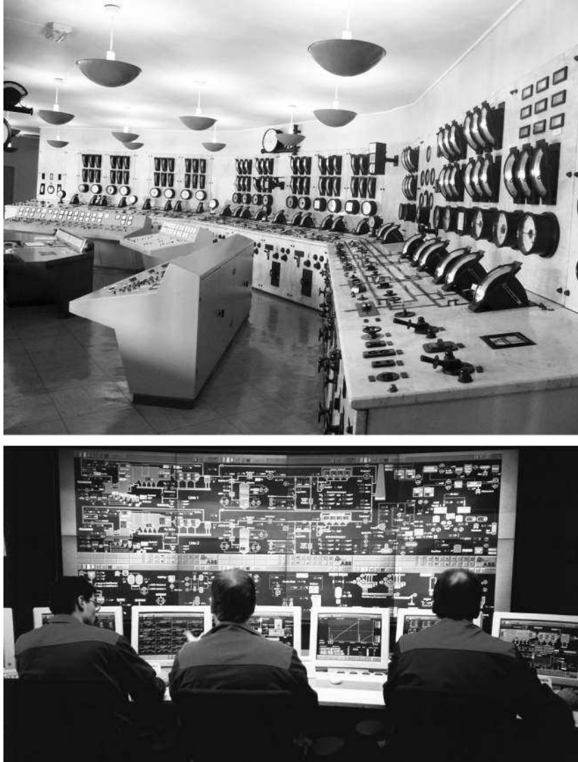
Figure 1.6 A control room of the 1960s and a more recent DCS control room (from Wikimedia Commons, the free media repository).
