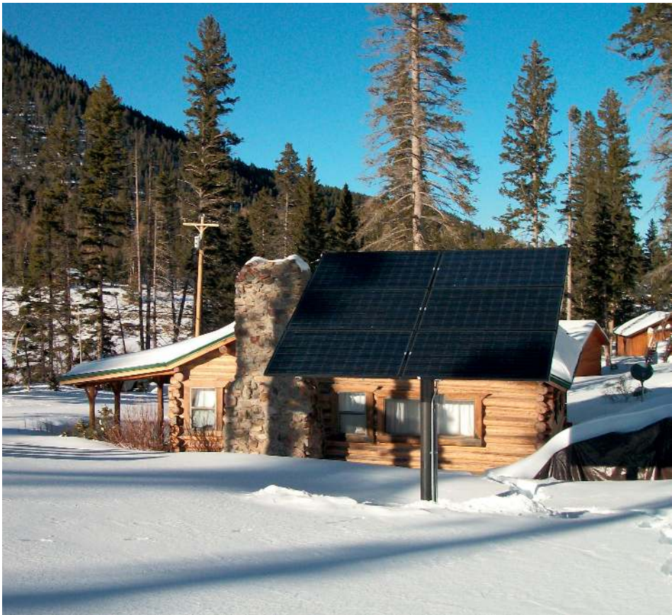
Figure 1.3 A solar photovoltaic array for a home in the state of New Mexico. There are six panels with a capacity of 190 W each. The array is connected to the electrical grid, which supplies electricity when the sun is not shining. When the array produces more electricity than needed, the electric cooperative buys the surplus. Solar arrays provide electricity without noise or air pollution. The solar panels themselves have become inexpensive, but there are substantial costs associated with the installation and integration into the grid. Germany has been the world leader in solar panel installations, with a capacity of 500 watts per person in 2017. Photograph by the author.
