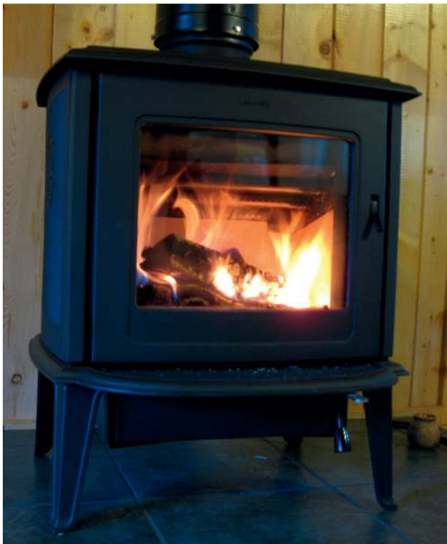
Figure 1.1 A wood stove for heating a home. This stove, manufactured by the Morso Company in Denmark, produces 6 kilowatts of heat. It has an efficiency of 75%, that is, only a quarter of the heat is lost up the chimney. There is a secondary pre-heated air supply at the top of the fire box that reduces air pollution by making the burn more complete. A wood stove can save money. A 6-kilowatt electric heater might cost a dollar an hour to run. However, it is hard work to saw and split the wood. Photograph by the author.
