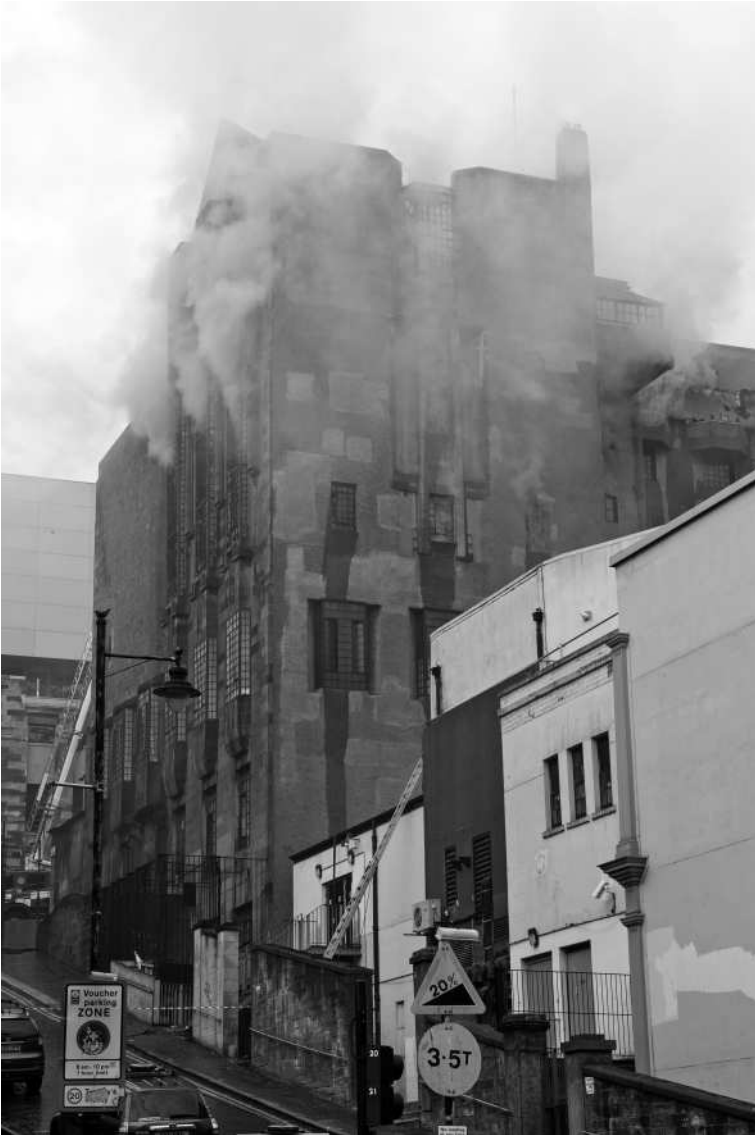
Figure 1 View showing the fire damaged south-west corner of the Mackintosh Building.
