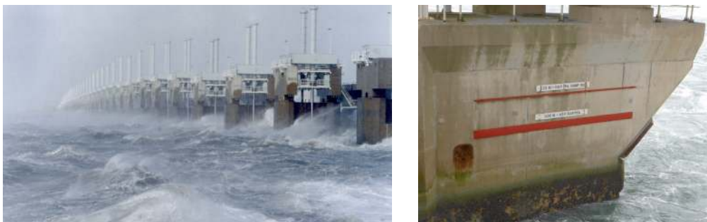
Figure 1.6 Left: The Oosterscheldekering at Neeltje Jans. Right: Its 3 m and 4.20 m storm-surge markers. Sources: Watersnoodmuseum (left) and authors (right)
