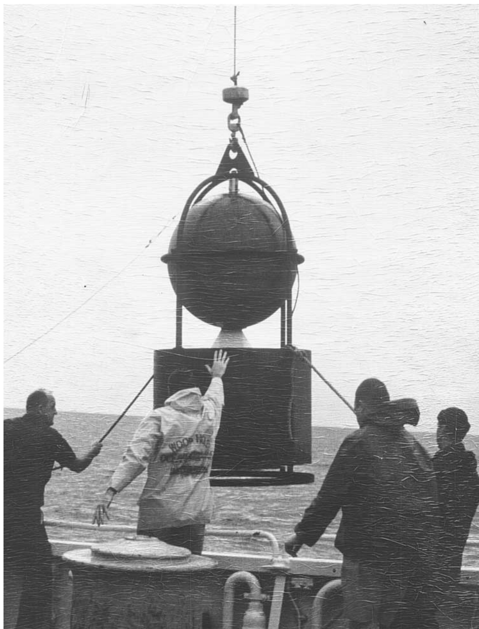
Figure 1.5 The aluminum sphere SOFAR float with the transducer underneath (mostly concealed by launch frame). See Plate 1 for color version.
