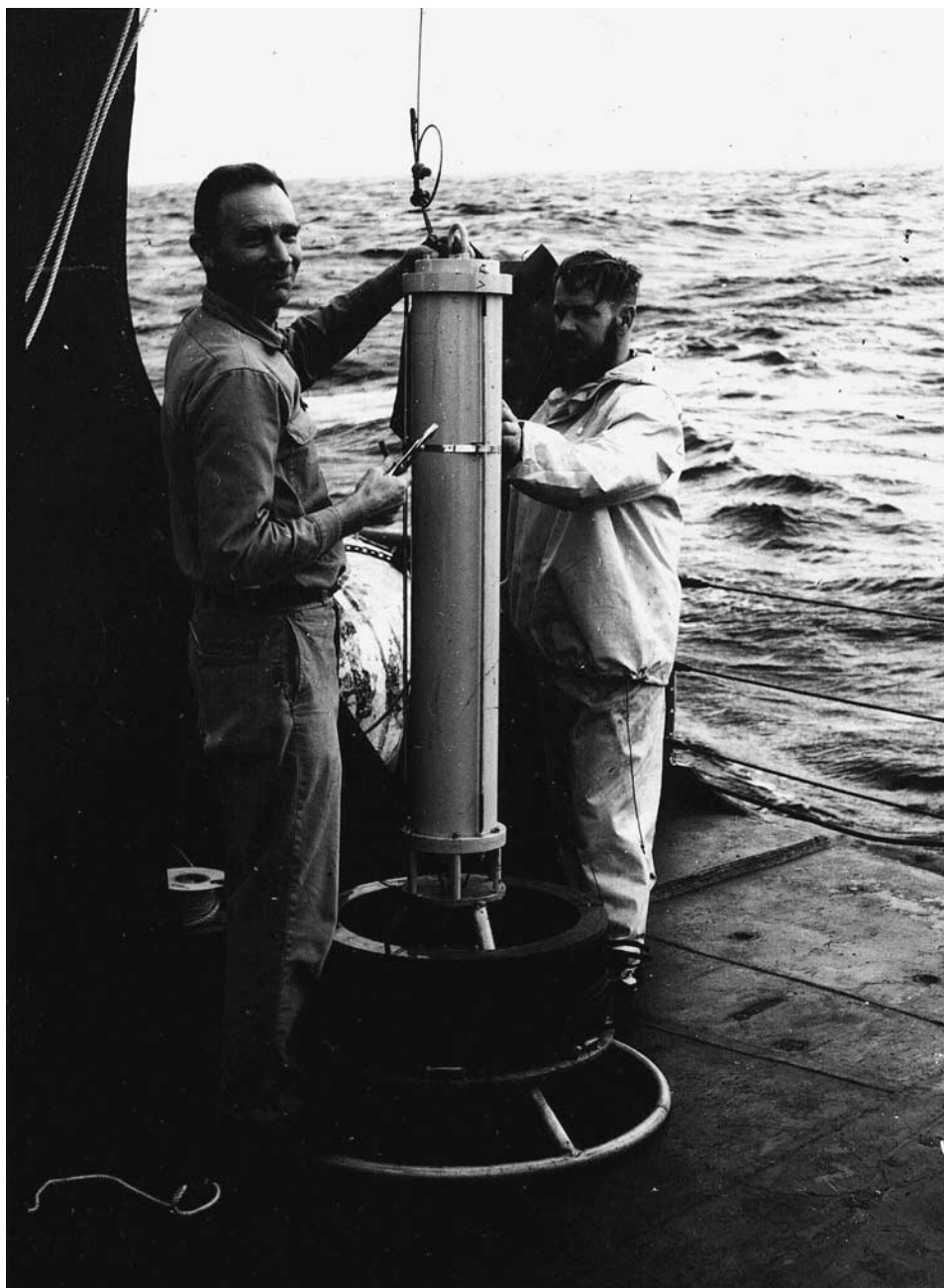
Figure 1.3 Gordon Volkmann (left) with acoustic transducer about to be lowered to sound channel depth to test long-range transmission through the ocean. The ring transducer visible below the shiny electronics module operated at 778 Hz.
