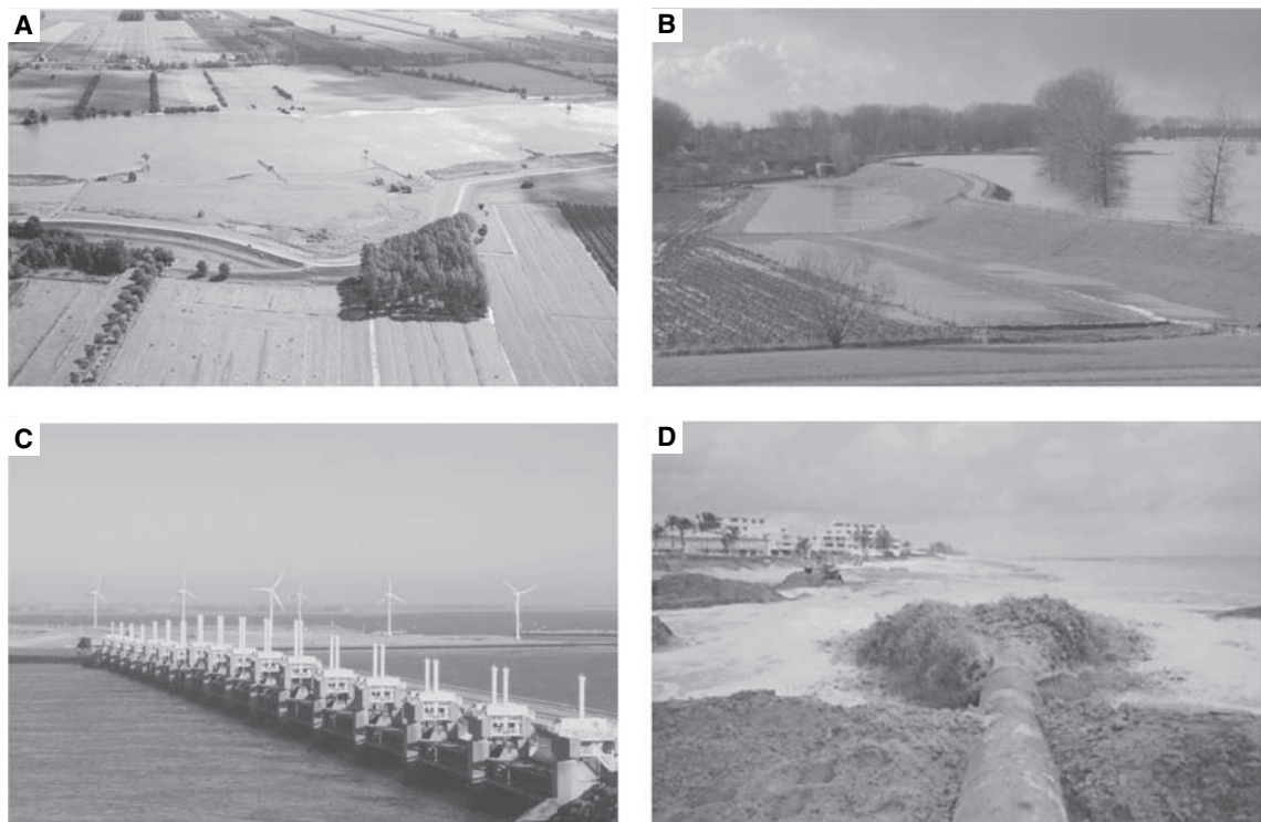
FIGURE 1.4. (A), (B) River engineering in the Netherlands: levees and groins. Photos courtesy of Henk Berendsen. (C) The storm surge barrier across the Oosterschelde Estuary, Netherlands. Photo courtesy of Robert Hoeksema. (D) Beach replenishment in Palm Beach County, Florida. Photo from http://www.pbcgov.com/erm/enhancement/nourishment.asp . (See Plate 4 for color versions.)
