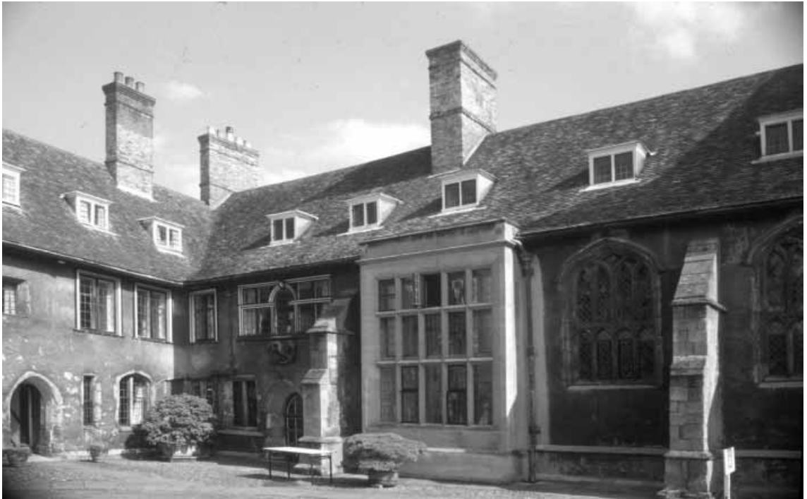
The earliest part of the College buildings. This picture shows the 14th-century structure, together with alterations in every century since.
