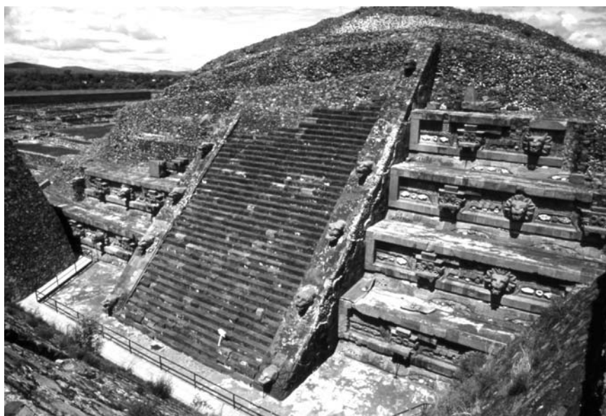
Fig. 3 Principal facade of the FSP. Photo: author.
