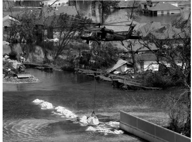
Figure 1.2. Failure of 17th Street Canal flood wall and catastrophic flooding of New Orleans, Louisiana associated with Hurricanes Katrina and Rita in 2005. The event received global attention and resulted in swift upgrades to New Orleans' long neglected flood control system. The broader influence of the event on US flood management is more incremental than paradigm changing. (Photo source: U.S. Army Corp of Engineers.)
