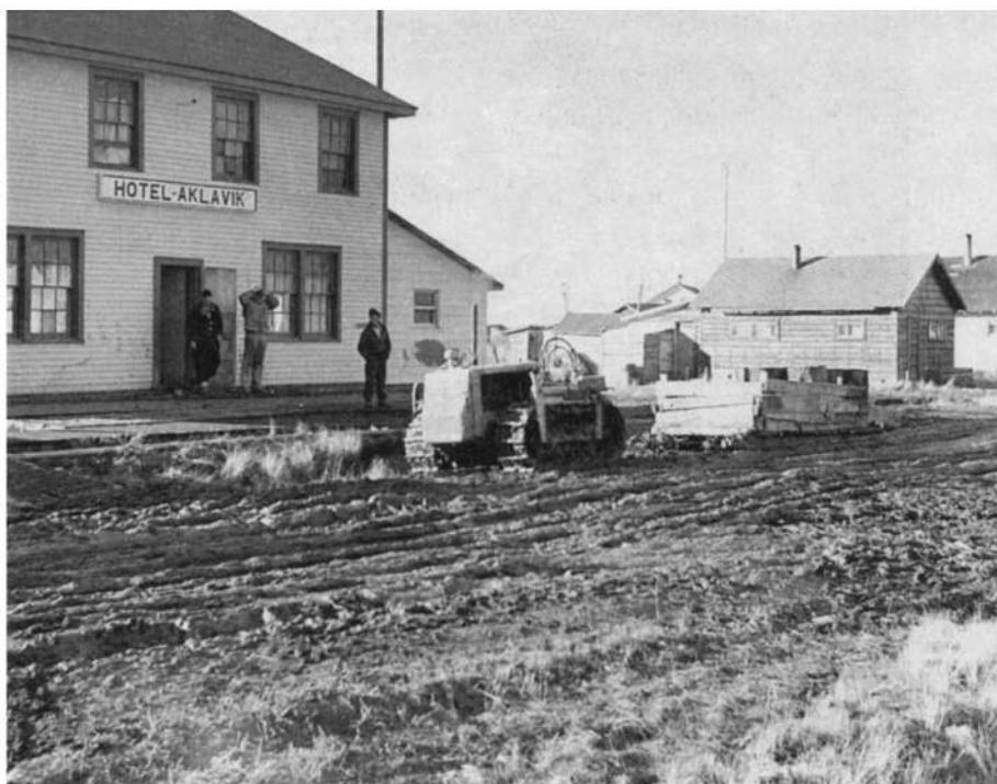
Figure 1.2 Aklavik. Northwest Territories. Canada, 1957. Thawing of frost heaved material, with drainage impeded by permafrost, resulted in roads being impassable for wheeled vehicles every summer. Modern construction methods, based on an understanding of the freeze–thaw processes, overcome this problem. Photograph from Williams (1986).
