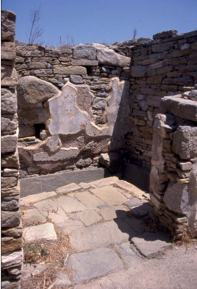
Figure 1.2 Toilet showing the paved floor with the water channel behind. Delos, Hermes House.
