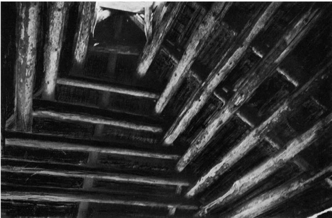
5 Summer cowshed: internal view to show construction of the pyramidal roof.
