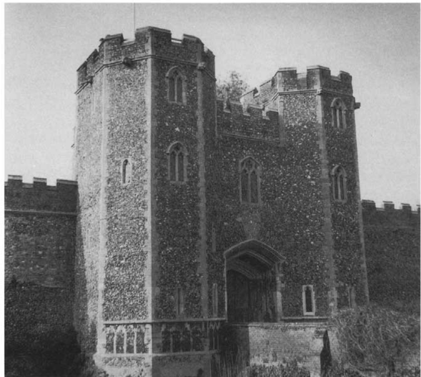
1 The gatehouse of fourteenth-century Wingfield Castle, Suffolk; although it has ornamental features like the flushwork and window tracery, the portcullis groove, arrow slits, moat and curtain wall on either side imply serious defence.
