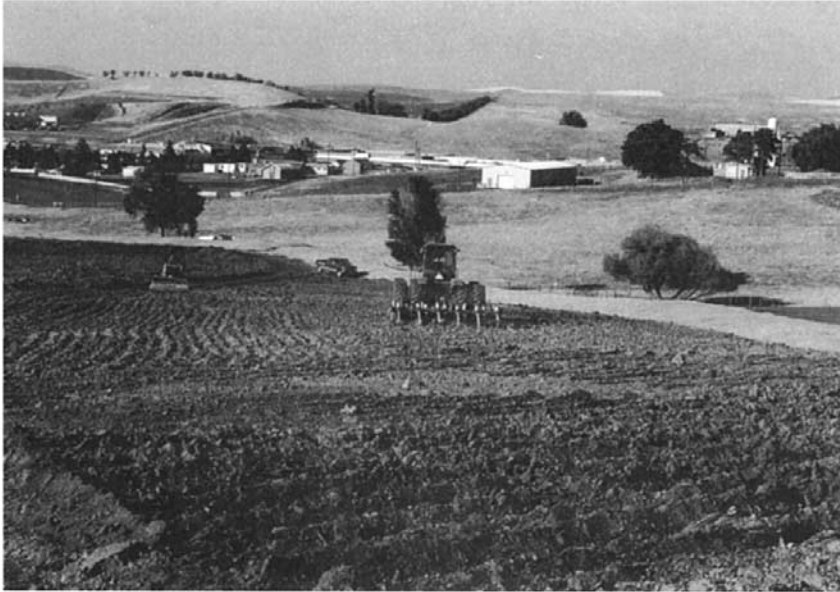
Figure 2. Landfarming of petroleum-contaminated soil. A 10-acre site for treatment of about 20 000 cubic yards of excavated soil.
