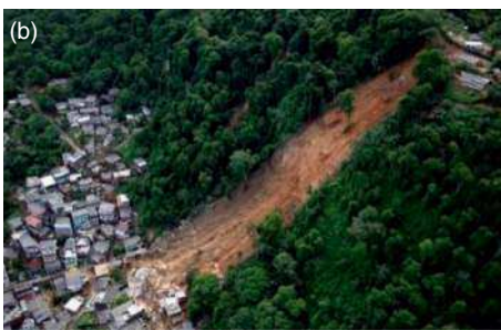
SCL Figure 8b Settlements on hillsides ( bairros-cota ); invaded areas belong to the Serra do Mar State Park. Such a settlement creates several hazards to its inhabitants, including landslides, floods, road accidents, and freshwater contamination.
