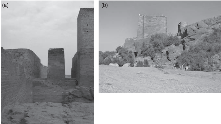
FIGURE 1.1. The Great Dam at Ma'rib. This massive waterwork was constructed and reconstructed over more than 1,300 years. It spanned more than 600 m between bedrock outcrops and stood approximately 19 m high. Rather than impounding water, the north sluice (shown left, as recently reconstructed by a German team) and south sluice (shown right) at the dam's extremities diverted water into an extensive series of primary, secondary, and tertiary canals that irrigated as much as 9,600 hectares (photos by the author).
