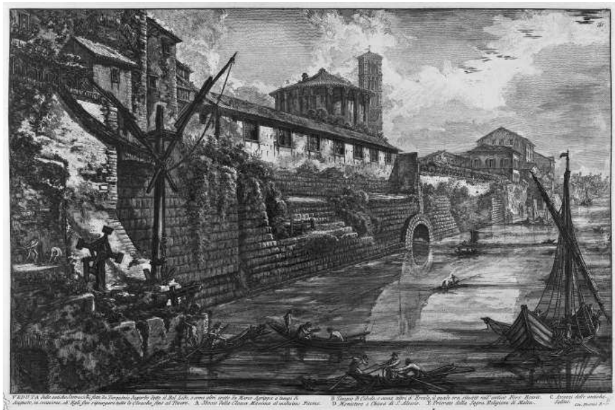
3. View of ancient Tiber embankment in mid-eighteenth century with mouth of Cloaca Maxima. Source: Piranesi 1747–1778. Wikimedia Commons/PD-Art.
