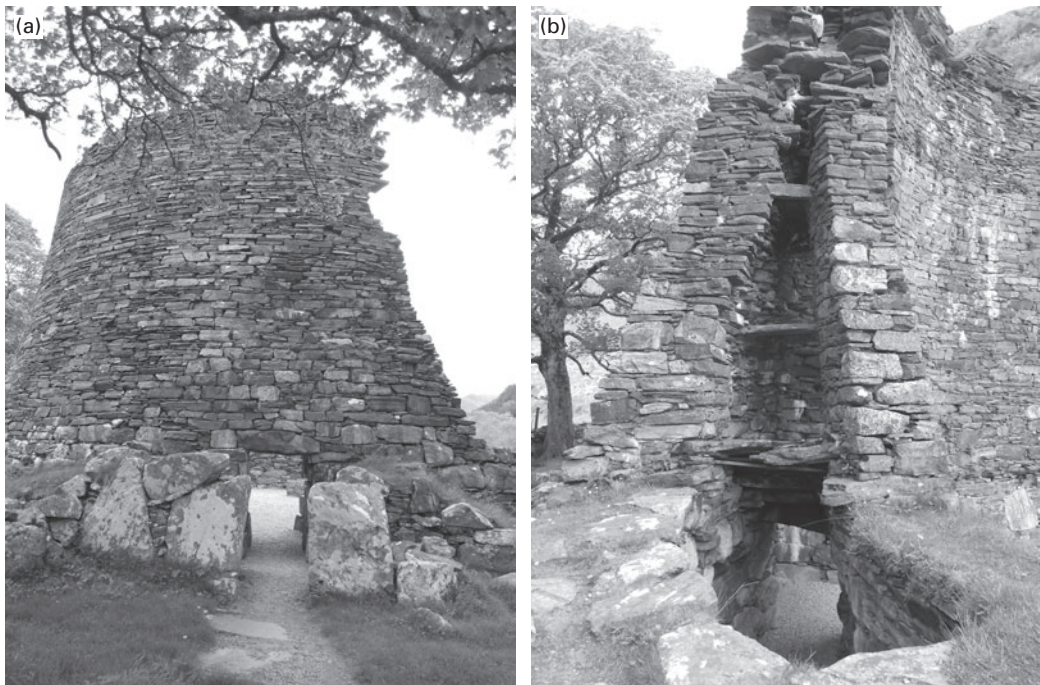
Figure 1.4. Remains of the fortified Iron Age farmstead or ‘broch’ of Dun Telve from Glenelg, Scotland (dated 500 BC to 100 AD), showing (a) the well-defended entrance and (b) the thick outer wall. Copyright of the author.
