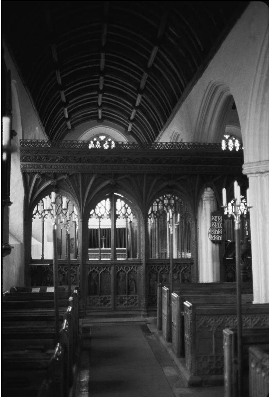
1 Rood screen: painted panels, windows, cornice. Ashton (Devon).
