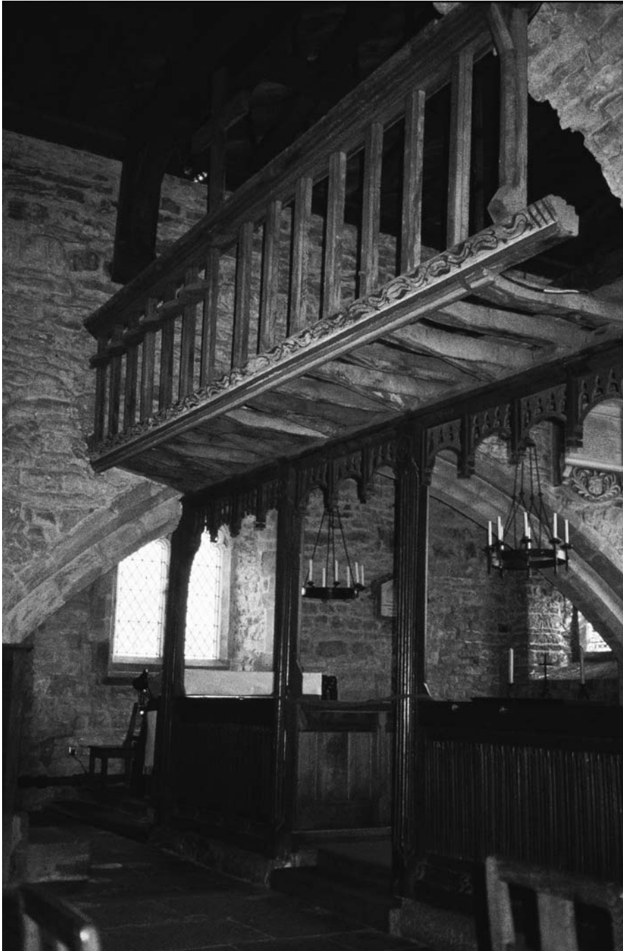
3 Rood screen and rood loft (1558): vacant niches. Hubberholme (Yorkshire).
