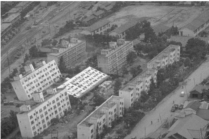
Figure 1.10. Failure of apartment blocks at Niigata, Japan as result of liquefaction induced by earthquake in 1964.
