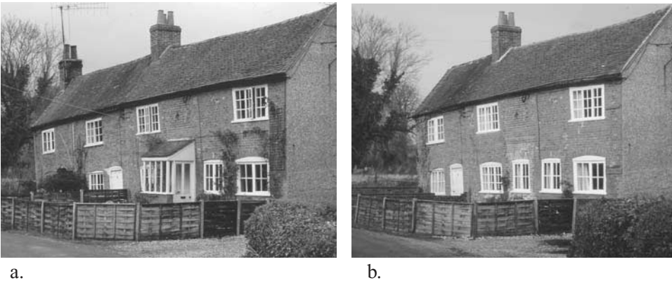
Figure 1.7. Row of cottages founded on soft ground: (a) before (1973) and (b) after collapse/demolition of end cottage (1977). (Stanford Dingley, UK).
