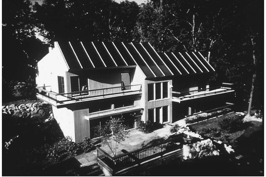
Figure 1.4 A domestic space heating collector. (Courtesy of the National Renewable Energy Laboratory, Boulder, CO.)
