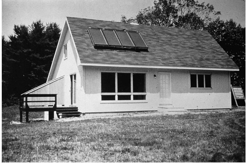
Figure 1.1 A solar domestic hot water (SDHW) collector. (Courtesy of the American Solar Energy Society.)
