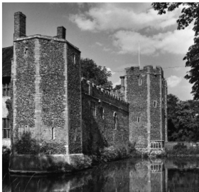
PLATE 3 Wingfield Castle: gatehouse and south-west tower
