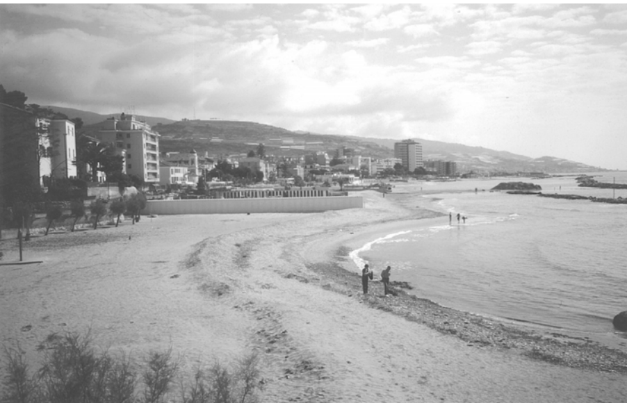
Figure 1.2 Arma di Taggia, Italy, showing onshore and offshore structures and beach grading operations that have changed the appearance and function of the coast by altering the energy of the waves, the topography of the beach and the natural vegetation and habitat.
